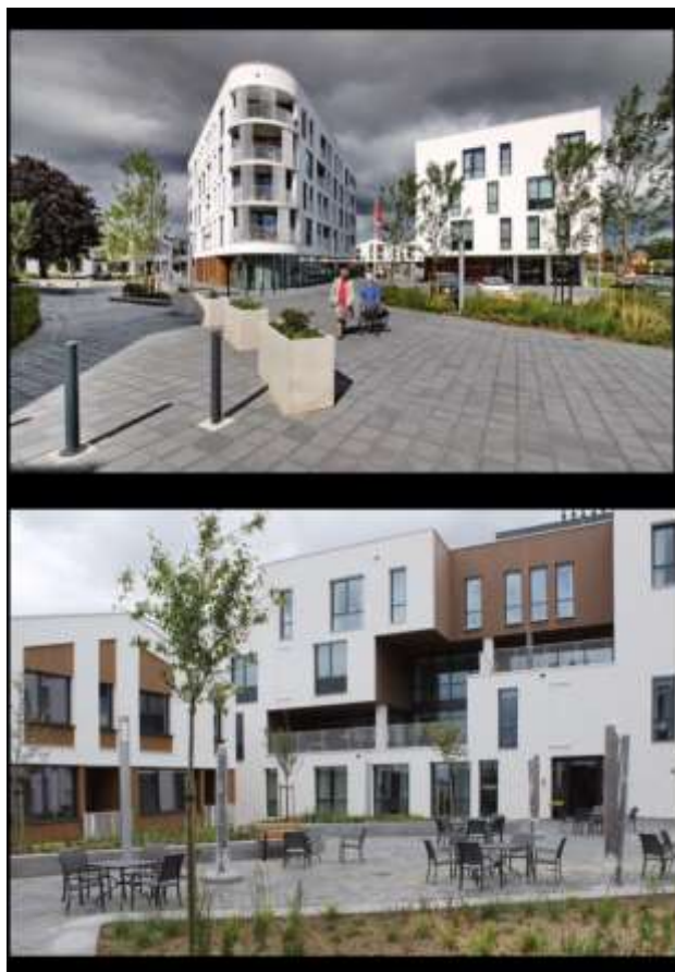
Plate 3: front and courtyard view of the hospital
