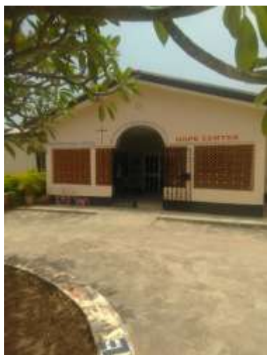
Plate 1: Approach view of Hope Centre Hope Centre
