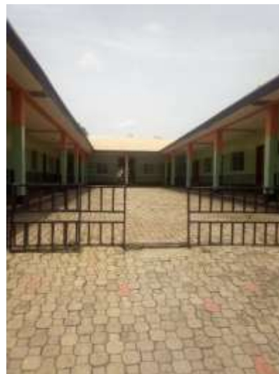
Plate 2: View of the Classrooms with courtyard at Hope Centre
