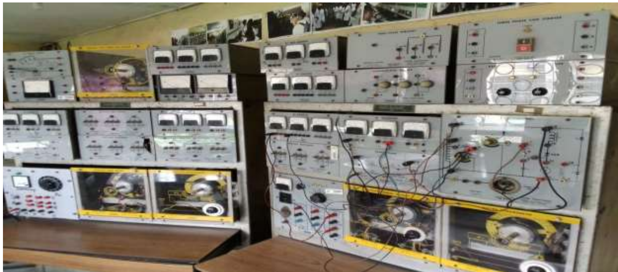
Figure 5: Research Laboratory with DC machine SCR [UNIPOINT]
