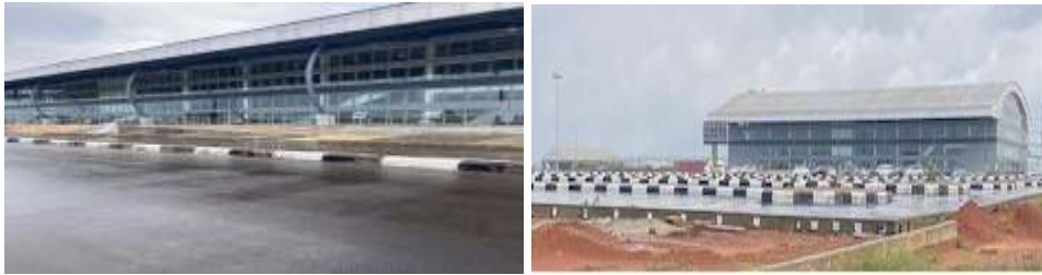
(Plate 1) Proper noise control within the terminal building using thick plate glazing and aluminum frames. Adequate passenger flow through the separation of departure and arrival passengers within the domestic and international area
