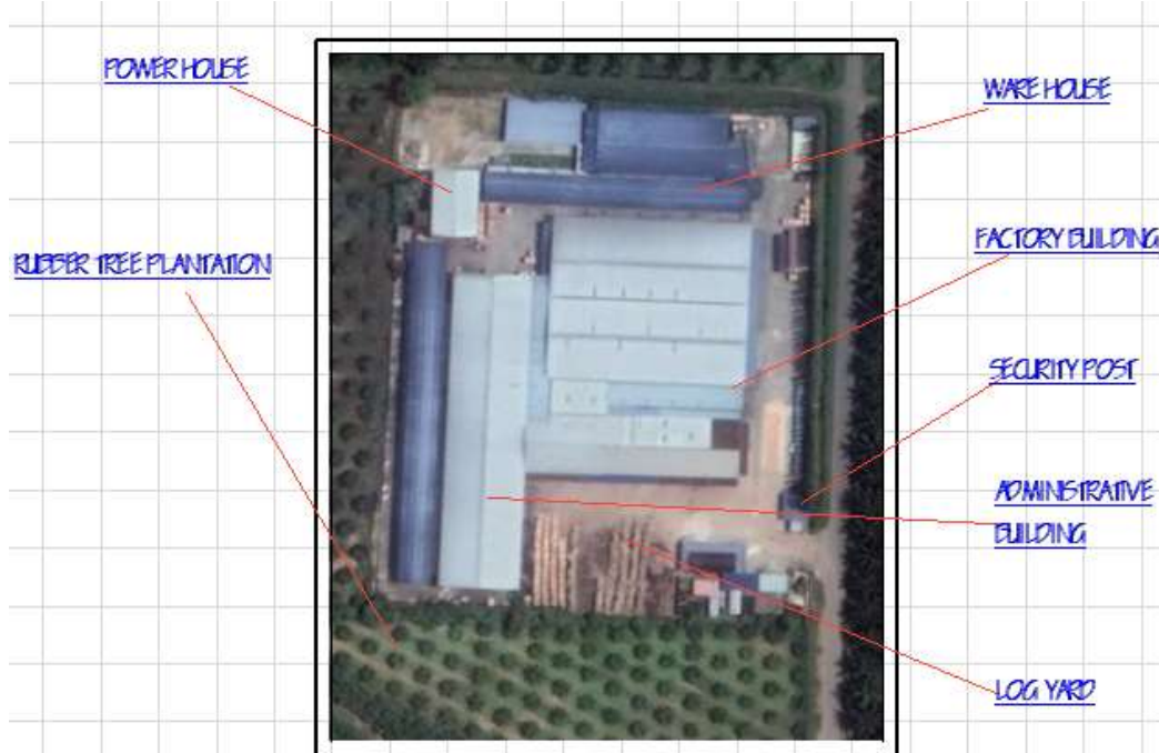
Plate 3: Site Aerial view of Ban Huat Rubberwood processing factory at Kedah, Malaysia Source: google earth, 2022
