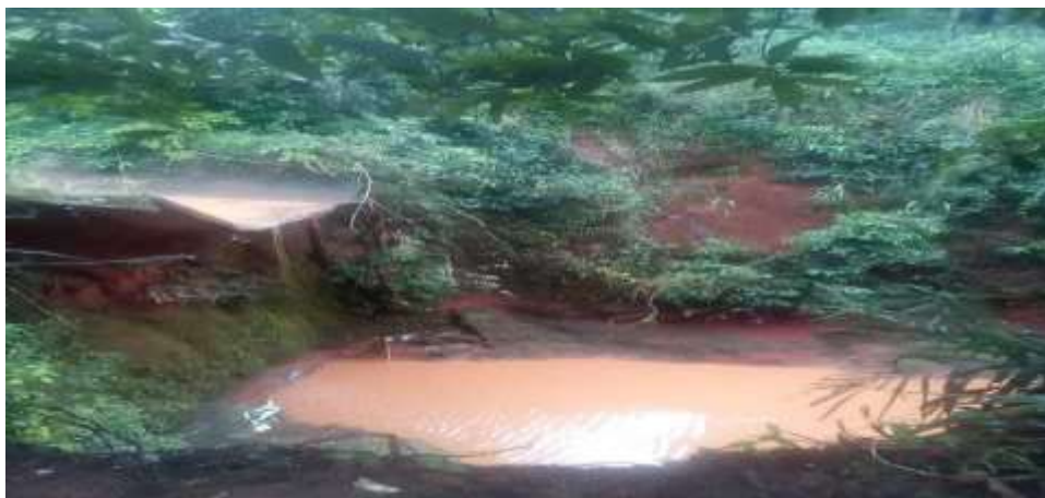
Obosi Erosion Site
