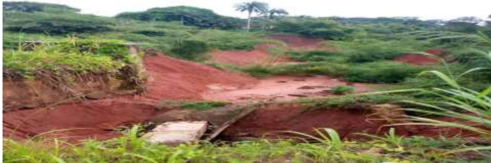
Erosion Site Achina
