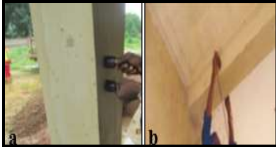
Fig. 3: testing the structural elements with PUNDIT, (a) ground floor column (b) first floor beam.
