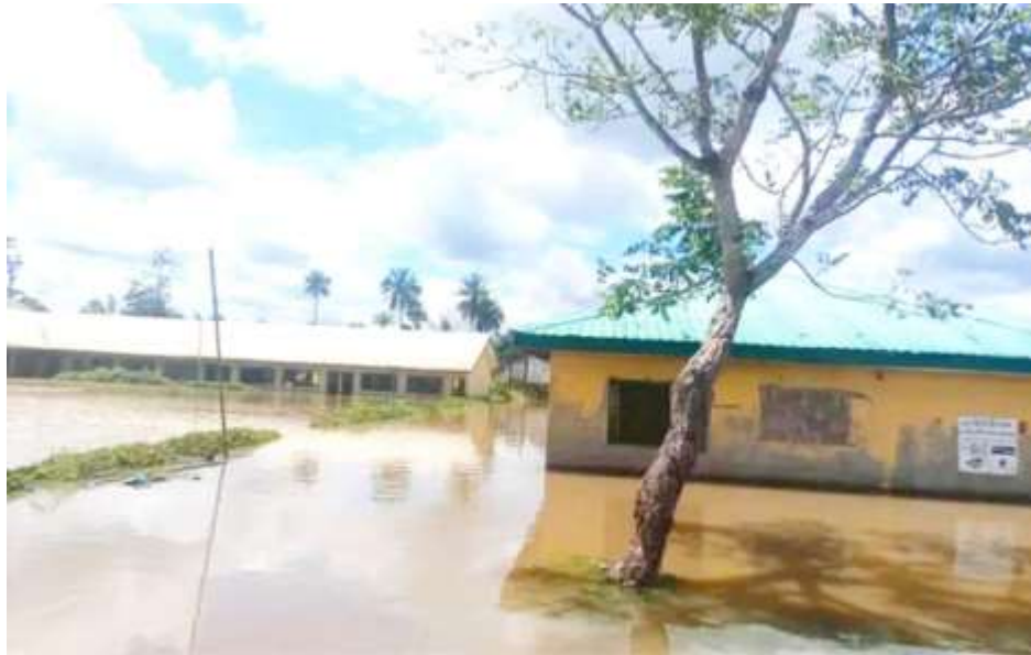
Figure 1 : Girls Secondary School, Kaiama, Kolokuma Opokuma LGA being overrun by flood water.
